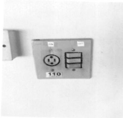
Interruptor e tomada
